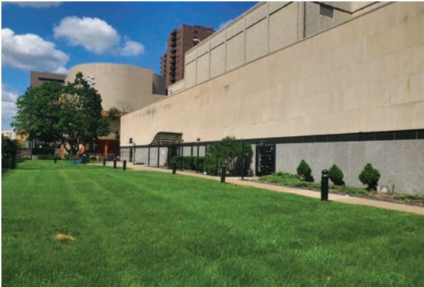
Front of building
